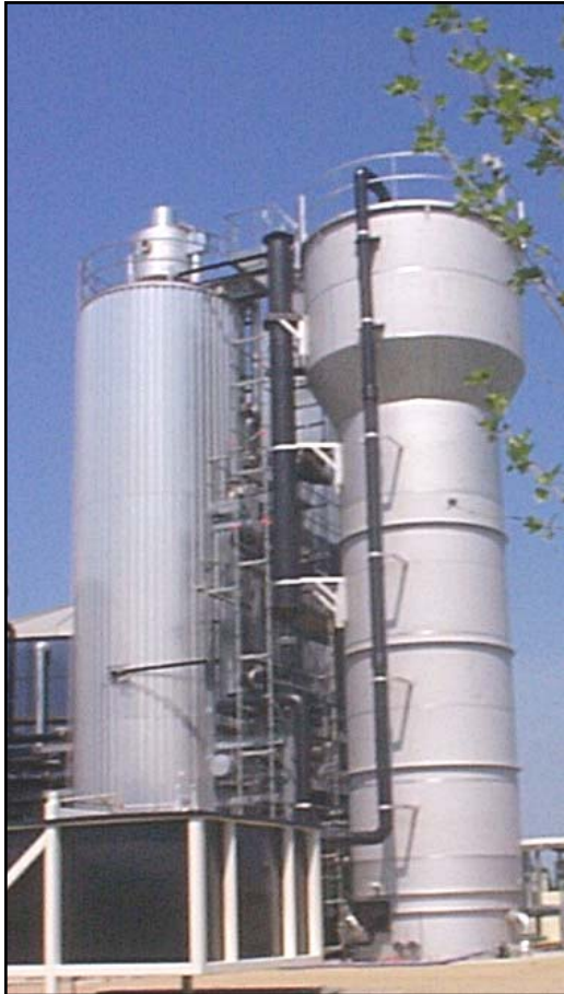
BIOPAQ -IC-Reactor
